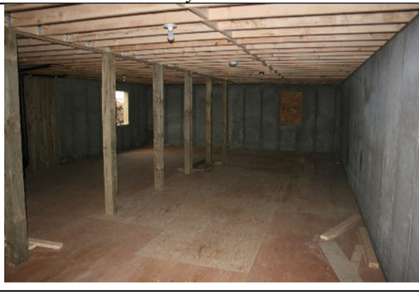
Riley basement area
